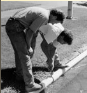
Above: Assembling a Certa-Lok Yelomine restrained joint. Top Right: Certa-Lok Yelomine's high impact strength and ultraviolet protection make it especially suitable for above-ground applications.
