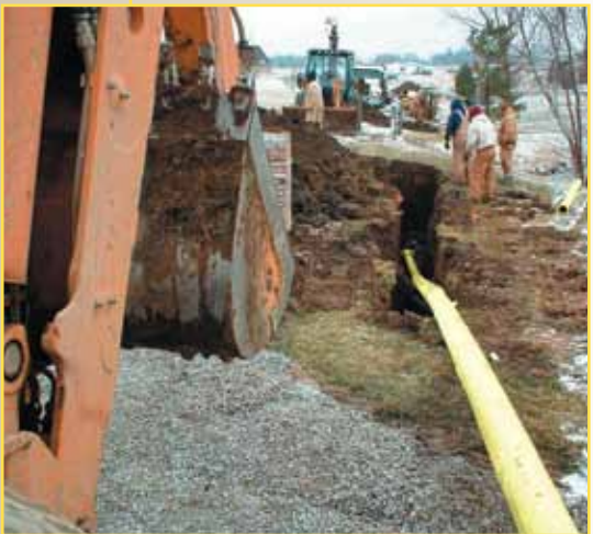
Yelomine IB trenchless installation
